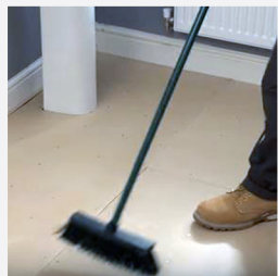
1. Preparation make sure the surface is free from any protruding objects
